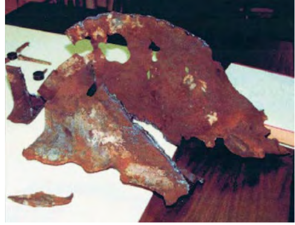
Figure 1.8 Steel from WTC 7 that experienced oxidation and sulfidation (FEMA, 2002).
